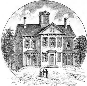
THE HIGH SCHOOL HOUSE. ERECTED IN 1851.
